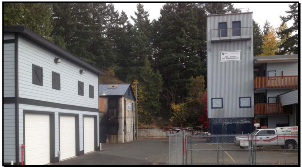
Comox Fire Training Centre
