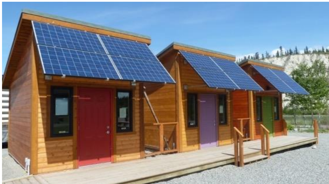
Pop-up business incubator workshops that are solarised could be temporary installations as part of an Arts Village on vacant parcels, or along the waterfront (Whitehorse, Yukon).
