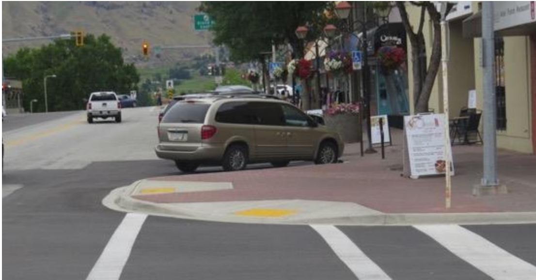
Existing Sidewalk Extension (bulge) on Main Street in Osoyoos.
