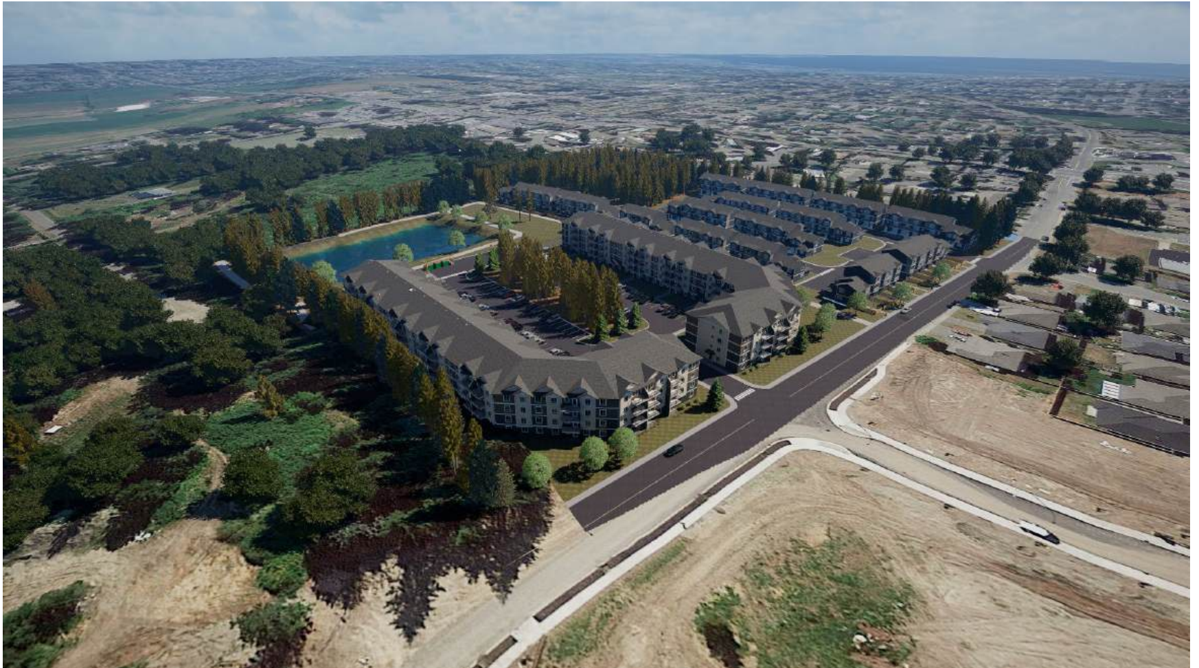
4-Storey Apartment Rental Units – Site View from Northwest to Southeast
