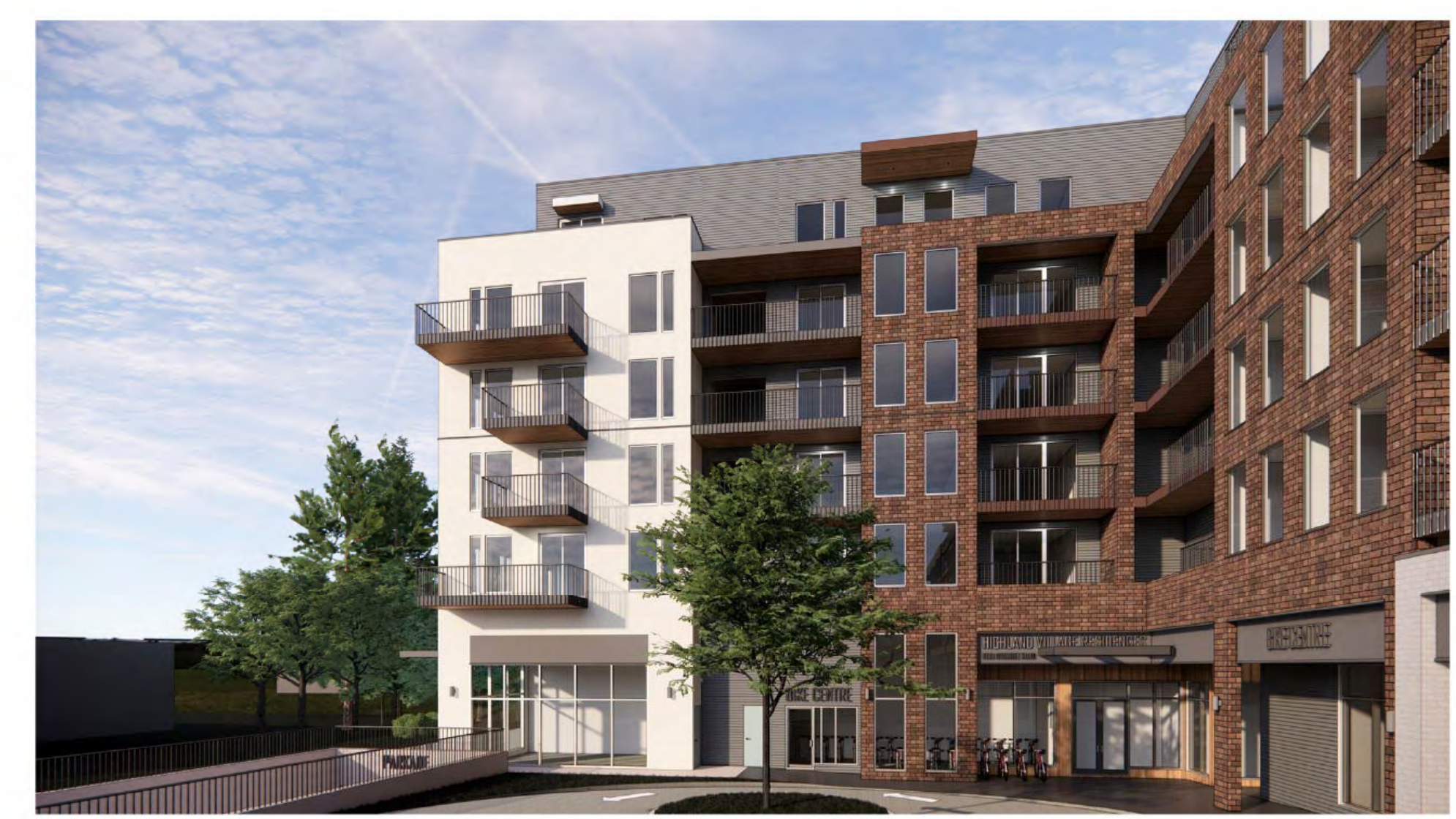
VIEW LOOKING AT THE RESIDENTIAL LOBBY ENTRANCE (NORTH VIEW)
