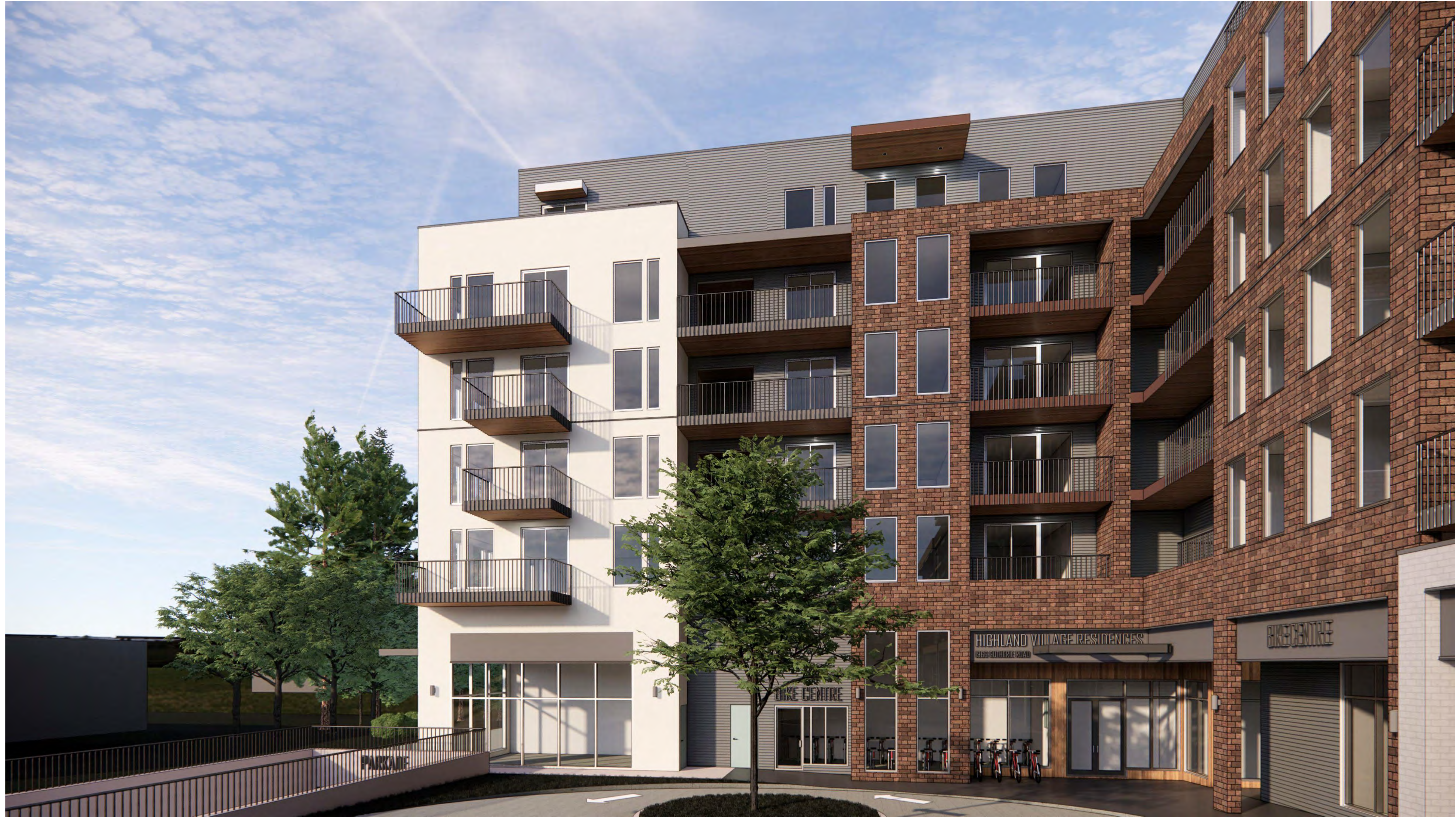
VIEW LOOKING AT THE RESIDENTIAL LOBBY ENTRANCE (NORTH VIEW)
